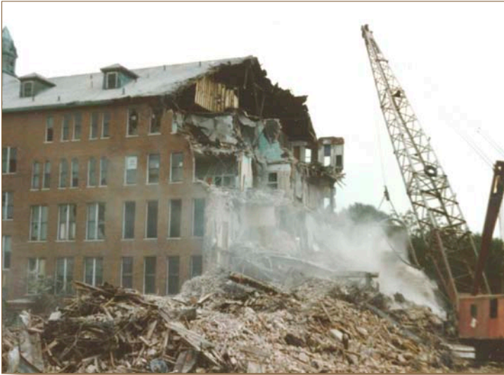
The demolition of the Sacred Heart Mission Seminary building.
