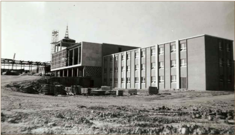
The new Divine Word College under construction.
