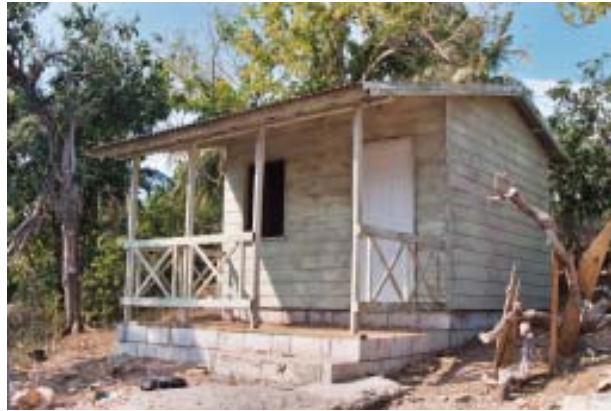
Alumni and crew completed this house in just five days! It is the new home to a single man who belongs to Our Lady of the Assumption Parish.
