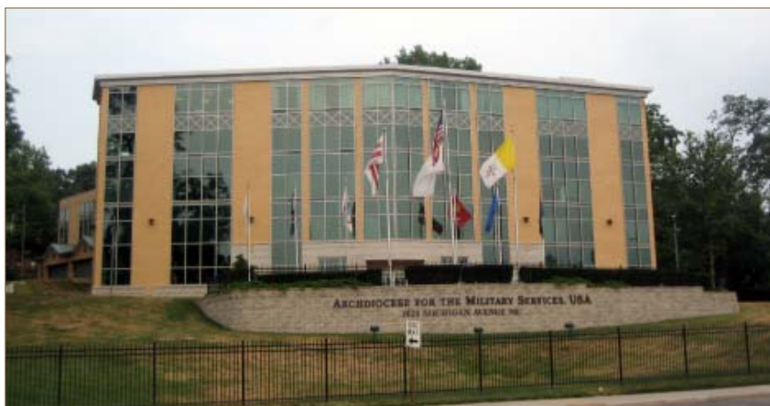
The Divine Word College Building as it looks today, the home of the Archdiocese for the Military Services, 1025 Michigan Avenue NE.
