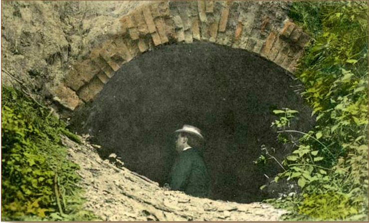
Tunnel entrance from Crosswicks Creek.
